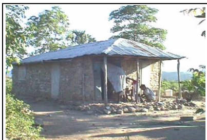
Figure 5 Tin-Roof house, Nan Labou, Diondion. Kitchen not visible
